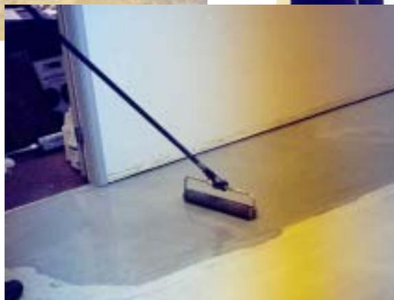
Polytop can be placed using a trowel or gauge rake to spread the material over the surface. A spiked roller can be used to remove any minor air bubbles that were created in the mixing of the product. A fresno trowel can be used to lightly finish the surface if desired.
