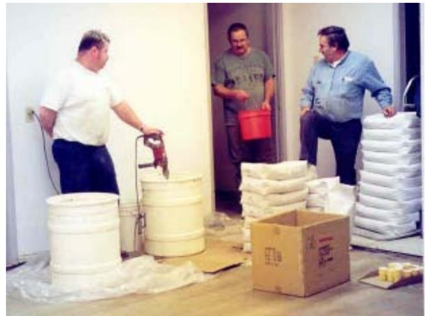
For small jobs Polytop is normally mixed in a 5 gallon plastic pail for one bag at a time or a 15-30 gallon drum where 3 - 4 bags may be mixed at a time. A mixing paddle with a 1/2" heavy duty electric drill with low speed 650 rpm is normally used.
