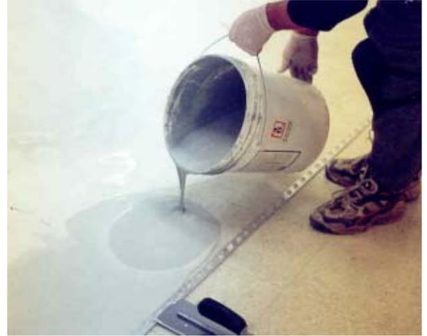
Polytop should be poured onto the surface and each subsequent pour should be placed in the wet edge to continue the flow of the material on the floor.
