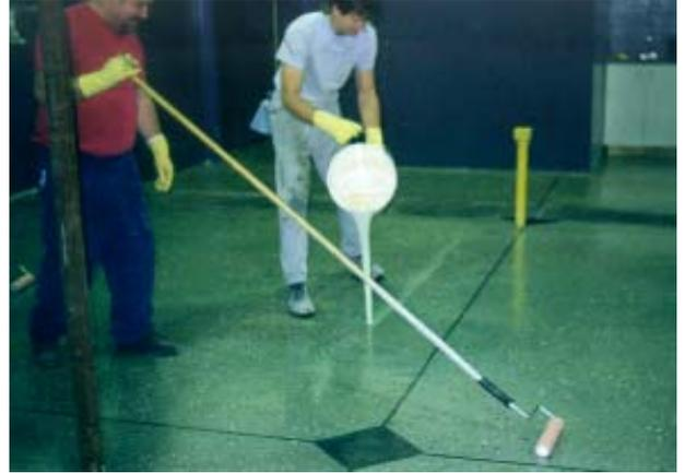
Epoxy or urethane sealers are normally used for indoor applications. Apply at 100 - 160 square feet per gallon using a low nap roller. Allow to cure for 3 days before application of the floor finish coat.
