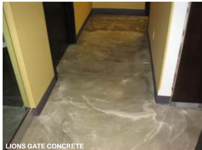
Spec-Deck improves the appearance of many surfaces. Spec-Deck can be applied in one or a combination of colours, smooth or textured, with an unlimited number of custom patterns. Your imagination is the only limit! Spec-Deck can be sprayed or trowelled, providing a stronger and more resilient surface than portland cement concrete. Spec-Deck is resistant to staining, water, salts and oils.
