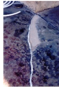
Backer rod inserted
