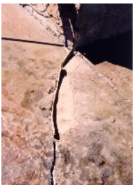
Repair done with form in place
