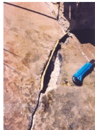
Cardboard form inserted ready for patching
