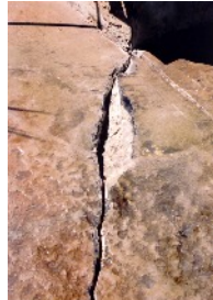
Concrete repair sawcut & cleaned up
