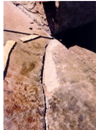
Form removed ready for sealant
